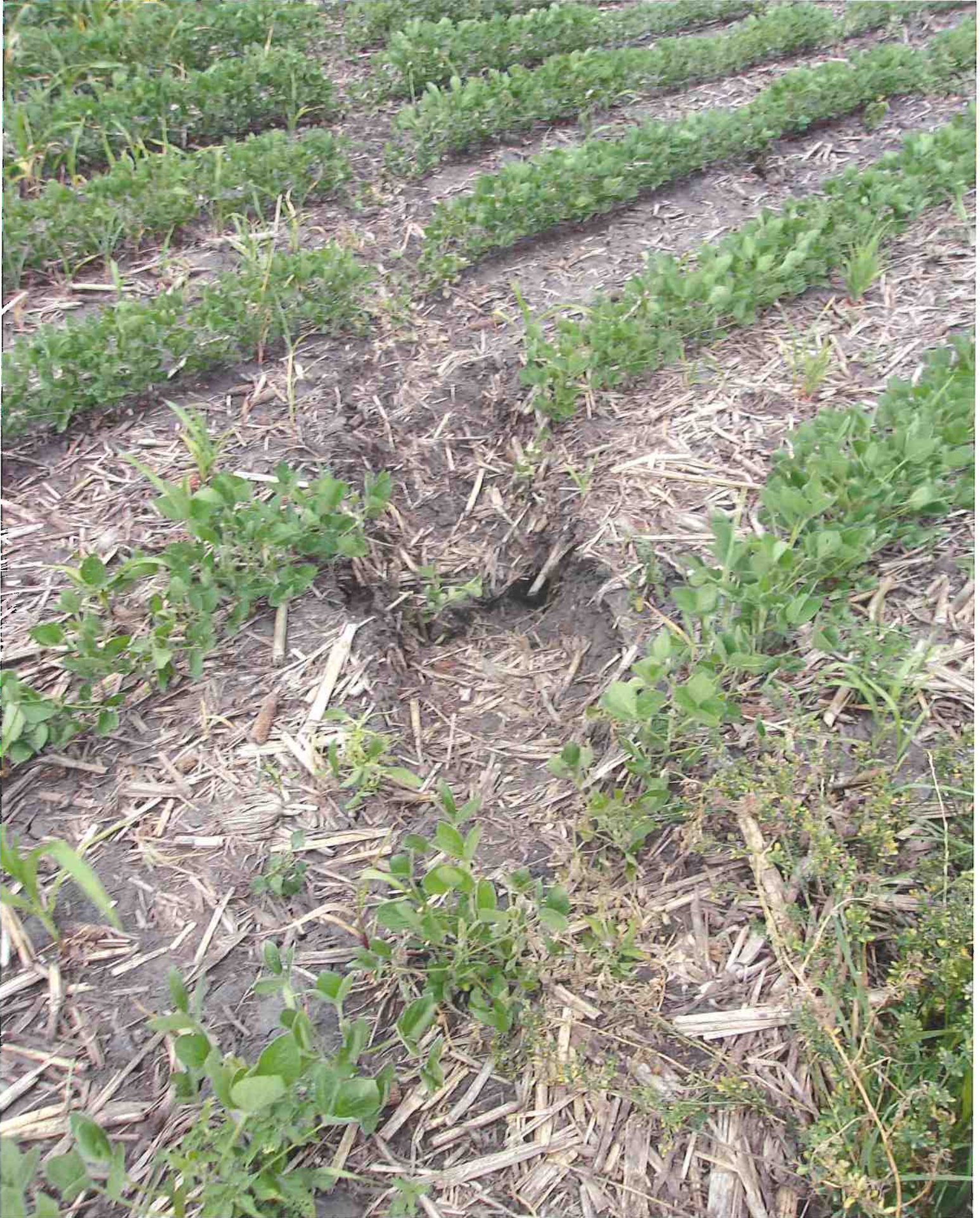
Collapsed Tile From Sprayer
